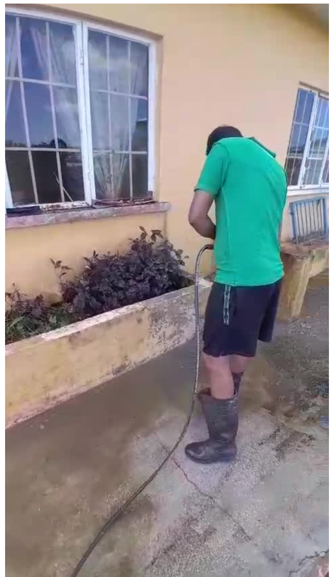
Walkways and external surfaces
