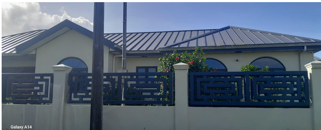
Daylight view of the roofline and exterior
