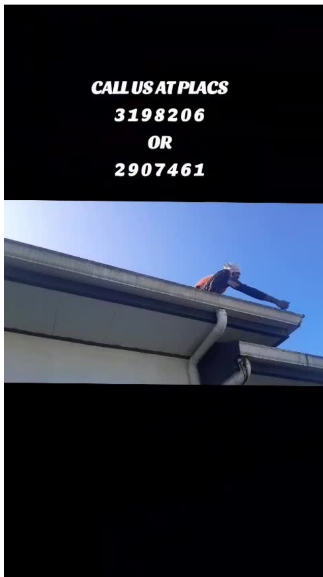
Roof cleaning in progress
