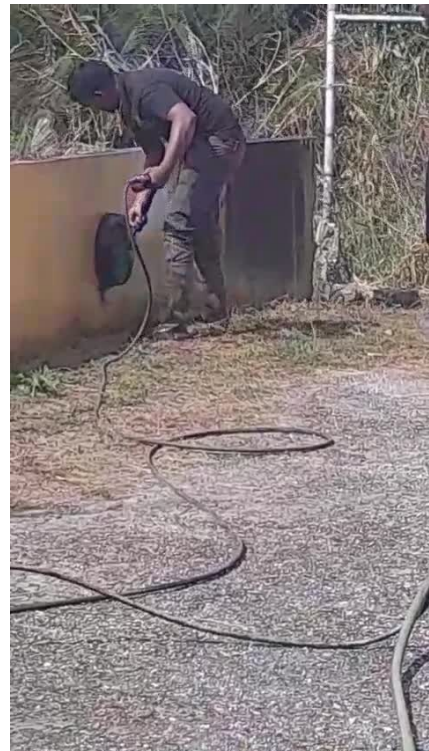
Wall cleaning in progress
