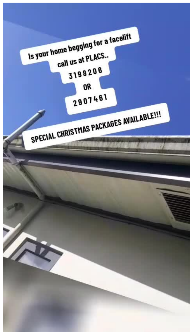
Roofline and guttering
